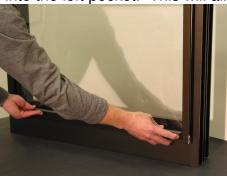
bring the prime sash out of the frame for removal.
