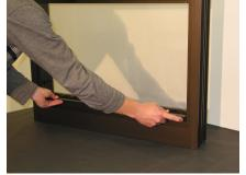
and release the pin-locks. The sash should stay in position.
