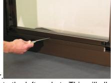
of the sill spacer. Lift upward and remove the spacer.
