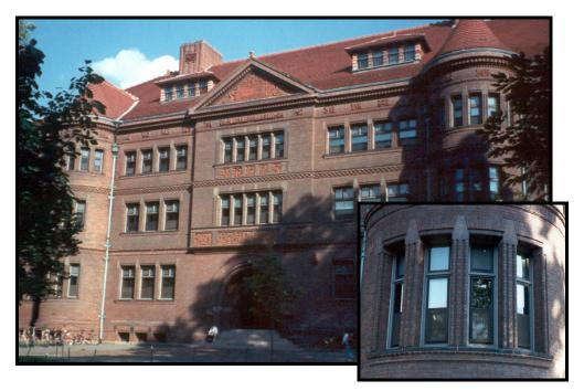
Sever Hall, in the heart of Harvard yard, was made more energy efficient by installation of new storm windows. However to avoid a "new" look for the building, the windows have a black anodized aluminum finish to retain the old traditional appearance of the building.
